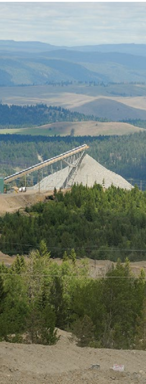
Courtesy of Copper Mountain Mining
