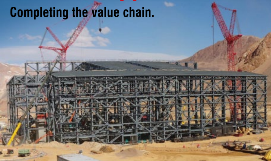
Construction begins on Barrick's Pascua Lama mill. It is expected to grind 45,000 mt/d starting in 2014. Photo courtesy of DIN S.A.
