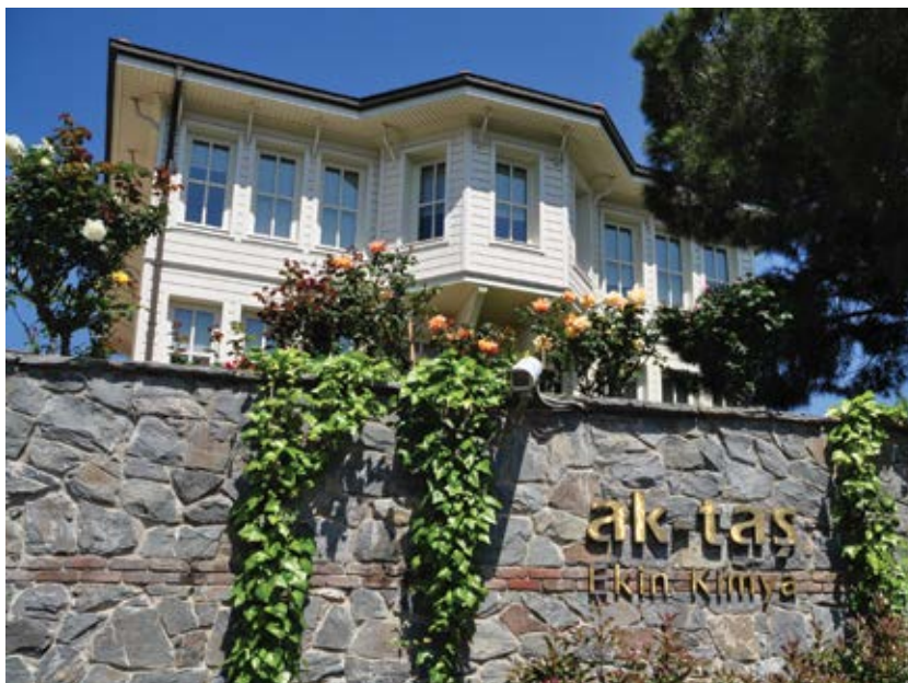
Ekin Kimya's headquarters in Istanbul. The firm has also established a new, 10,000 m 2 plant within the GEBKIM Organized Industrial Zone.
