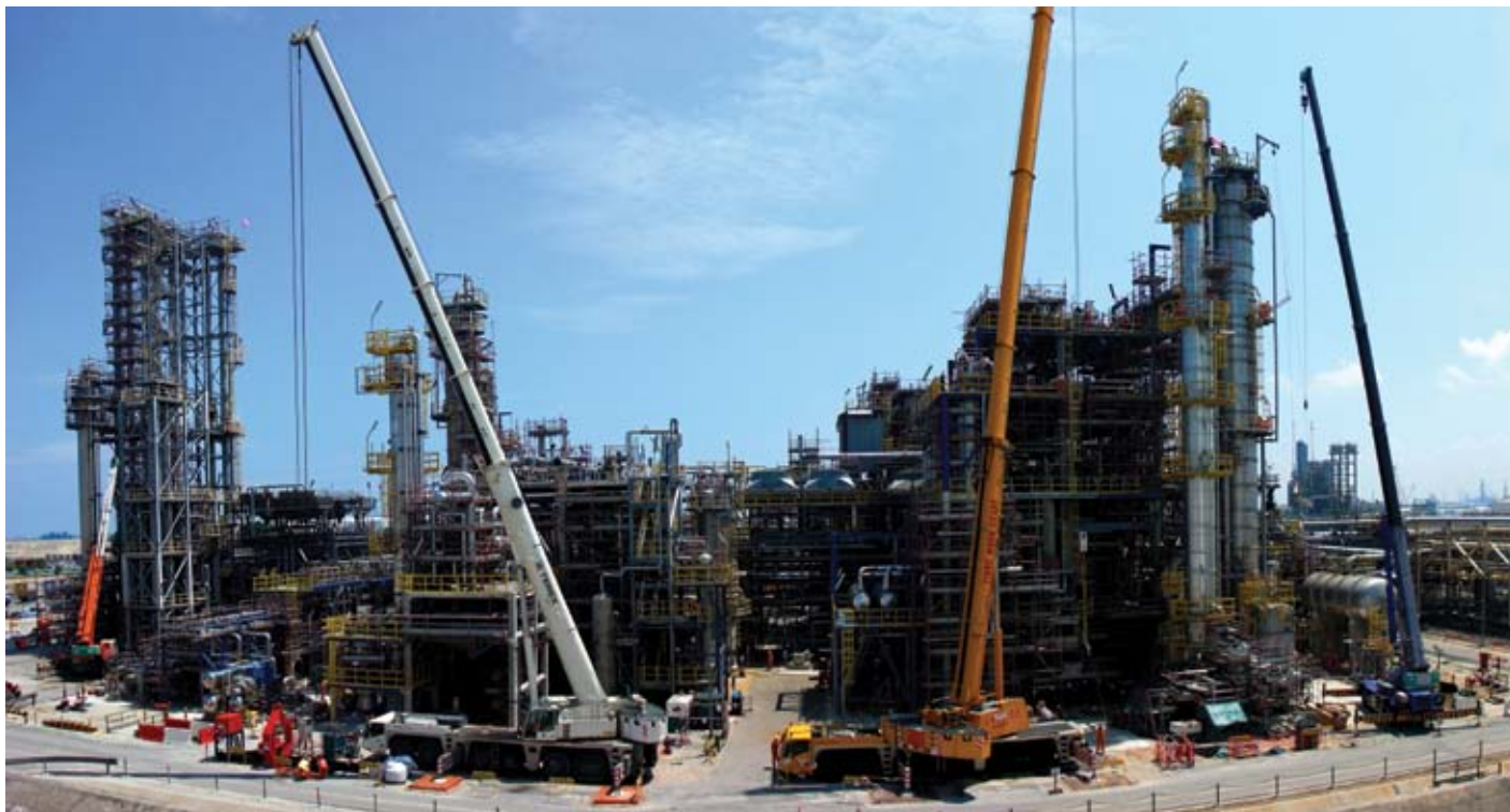
Material Installation by crane taken at the SPA-X Project (Singapore Alcohol Expansion Project) Photo Courtesy of McConnell Dowell
