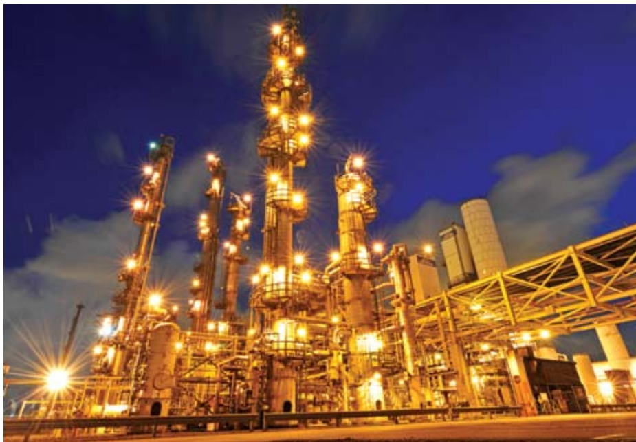
Linde Gas Singapore, Jurong Island plant
