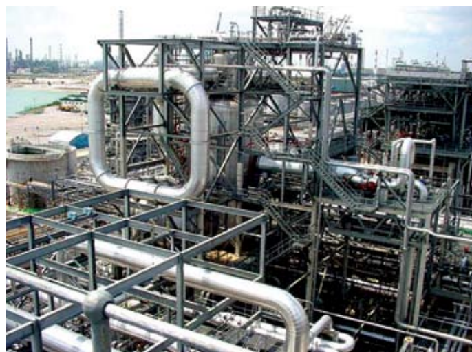
Structural steel. Photo courtesy of Hai Leck Engineering.
