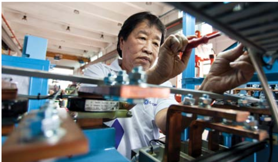
Control panels are designed and built in-house. Photo courtesy of Cyclect
