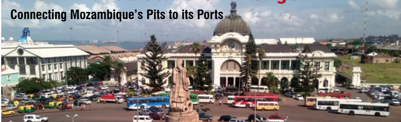
CFM central station. Photo courtesy of Tora Holding.
