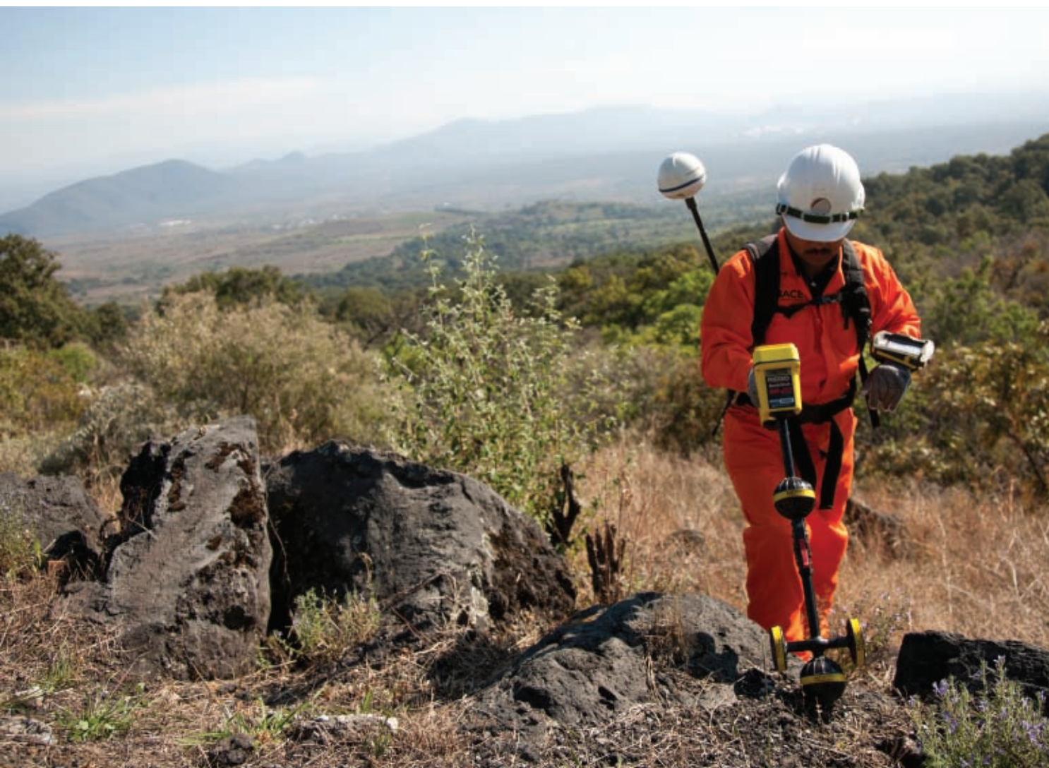
Stroke and Pipeline Location. Courtesy of Corrosion y Proteccion
