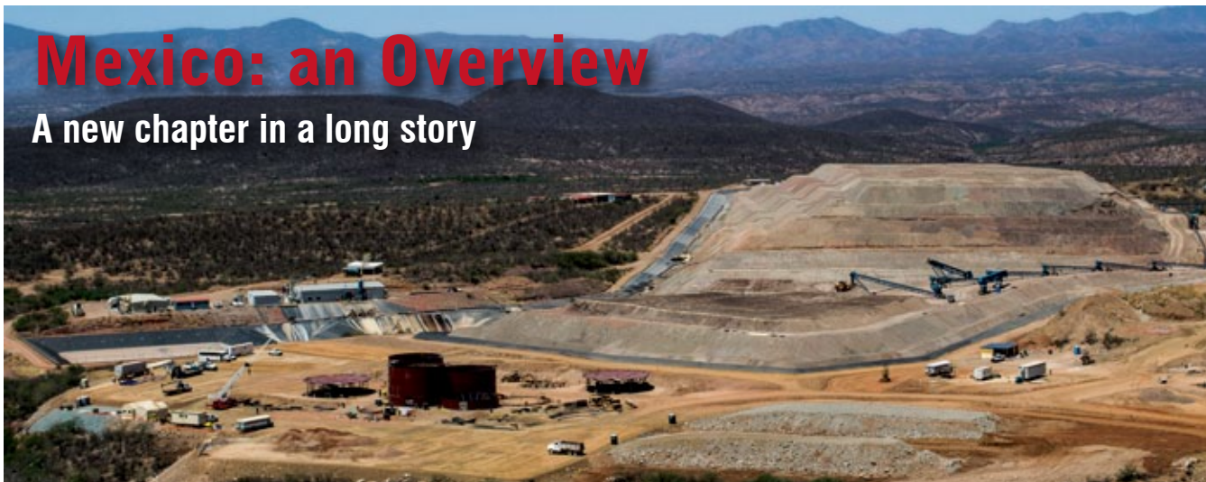
Santa Elena overview with original heap leach pad in the background, new heap leach pad, conveyor system and the new mill construction in the foreground. Photo courtesy of SilverCrest Mines.
