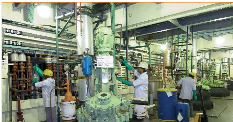
Inside Rubamin facility
