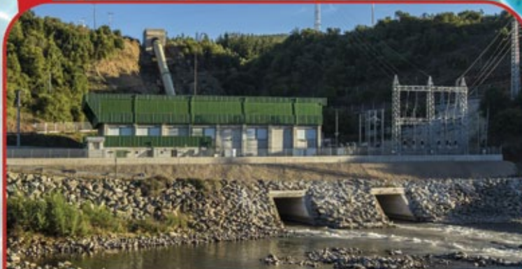
LIRCAY HYDROELECTRIC PLANT
