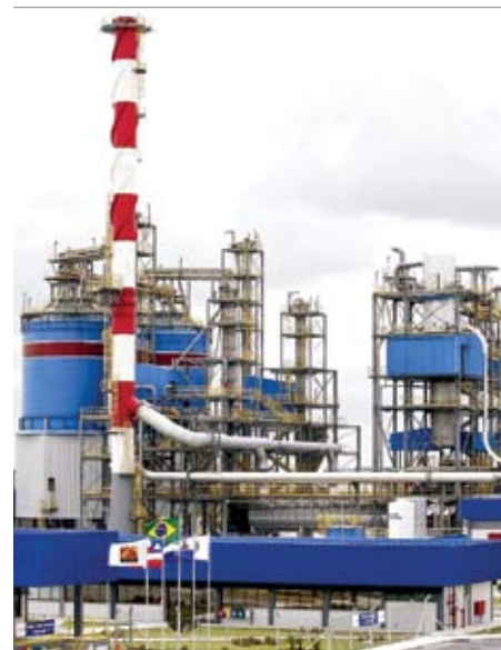
Birla Carbon operations at its Camacari Plant
