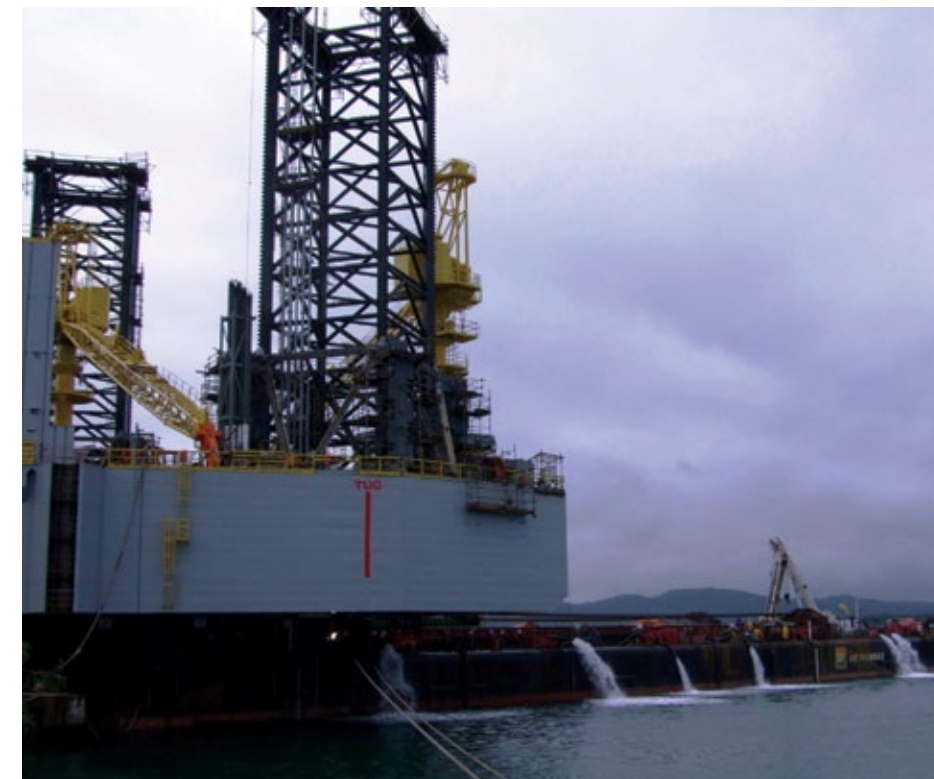
Load out of 6000 Te offshore platform onto barge at Bahia state, Brazil. Photo courtesy of Mammoet.
